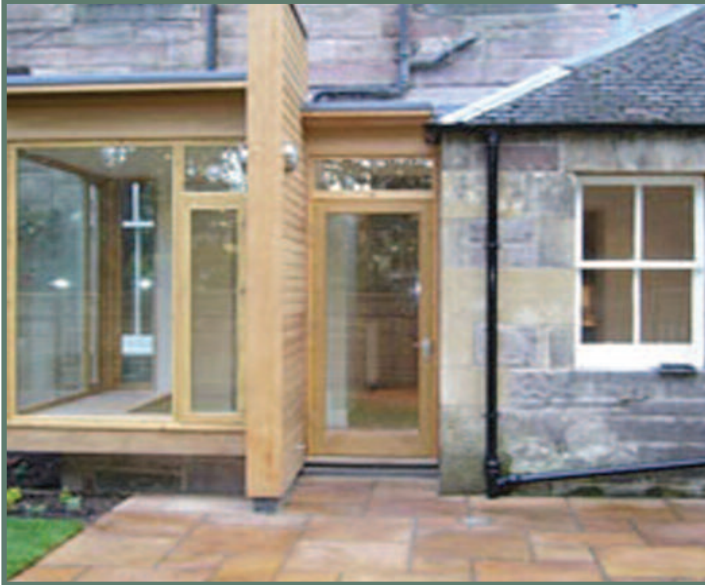
Marchmont Road transformation: "Too often the significance of the engineer's contribution is undervalued..."
