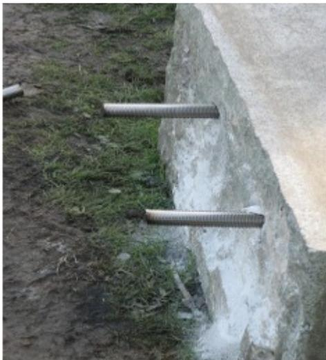
*Foundation stone drilled with stainless steel rods inserted*
