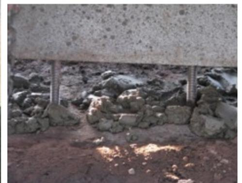
*Steel rods offered to drilled foundation on a bed of soft stabilising cement*
